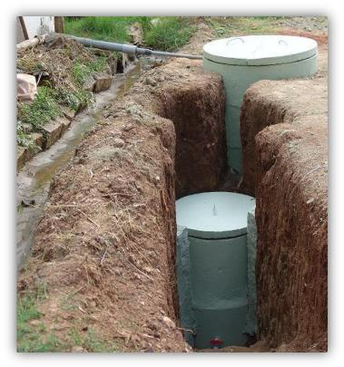
Bio-digester is used to convert organic wastes, insecticides and medicinal plants into a nutrient rich liquid bio-pest control.
